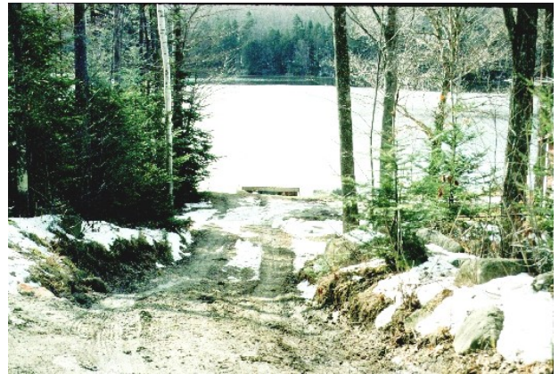
This driveway is sunken and eroding, running directly downhill toward the lake. Steps are needed to improve this situation to protect the lake from sediment pollution.
