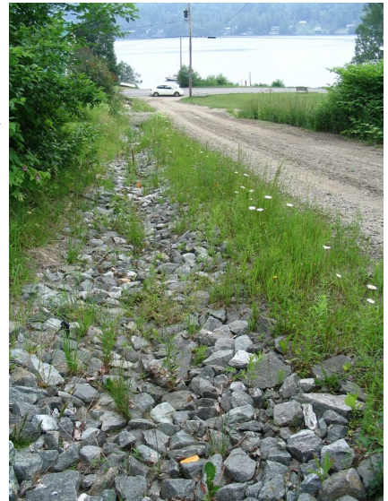
At left, lake association members seed and mulched a newly cleaned ditch. Center, rip rap stabilizes a culvert inlet area, often a site of either road edge erosion, or inlet pool erosion. At right, a steep road that serves several camps has had a rock lining installed to prevent the previous on-going erosion of the ditch.
