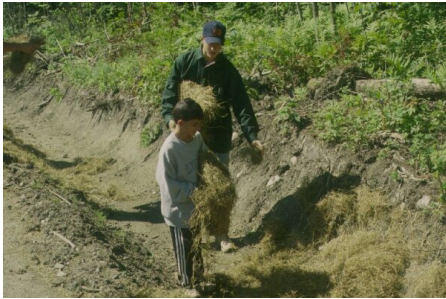
At left, lake association members seed and mulched a newly cleaned ditch. Center, rip rap stabilizes a culvert inlet area, often a site of either road edge erosion, or inlet pool erosion. At right, a steep road that serves several camps has had a rock lining installed to prevent the previous on-going erosion of the ditch.
