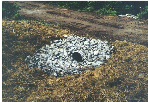
At left, lake association members seed and mulched a newly cleaned ditch. Center, rip rap stabilizes a culvert inlet area, often a site of either road edge erosion, or inlet pool erosion. At right, a steep road that serves several camps has had a rock lining installed to prevent the previous on-going erosion of the ditch.
