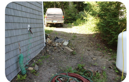
A steep slope site. Above 12% slope.
