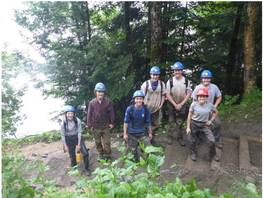
Northwoods Stewardship crew working on infiltration steps on Seymour Lake. Infiltration steps prevent erosion on walkways leading to the lake, and is one of the many Best Management Practices utilized along shorelines. NWSC crews have Erosion Control Certificates.
